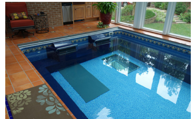
Fully In-Ground Indoor Installation
